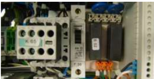
Secondary fuse isolation transformer 1-pole B16A
