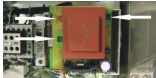
Fuses in cabinet for power supply unit
