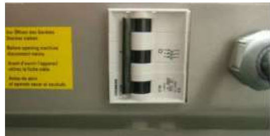
Expulsion fuse, device fuse 3-pole C16A
