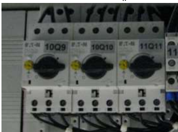
Motor circuit breaker
