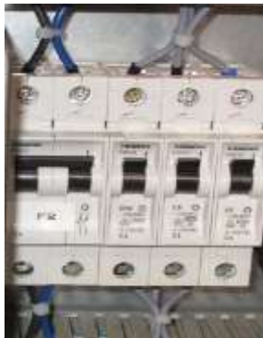
primary and secondary fuses
