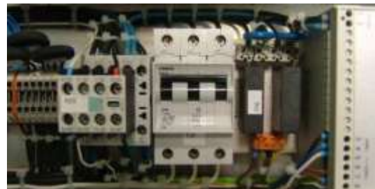
Secondary fuse isolation transformer 3-pole C16A
